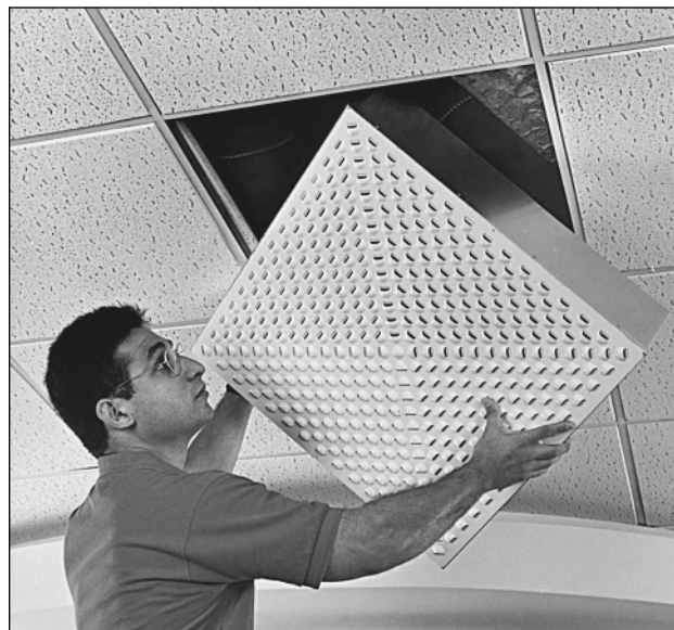
5 Technician installing a lay-in style of personal diffuser. This unit mixes supply air with room air by maintaining a fixed outlet velocity at reduced supply air flows. Photo courtesy of Warren Technology.
