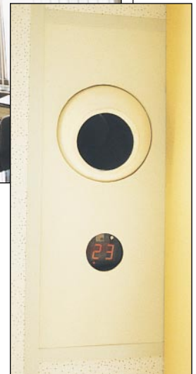
4 Personal diffuser installed in an office. This style provides air diffusion by injecting a stream of air into the room. Inset photo is a closeup of the diffuser. Photos courtesy of Zero Complaints.
