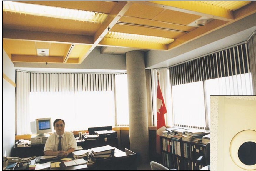
4 Personal diffuser installed in an office. This style provides air diffusion by injecting a stream of air into the room. Inset photo is a closeup of the diffuser. Photos courtesy of Zero Complaints.
